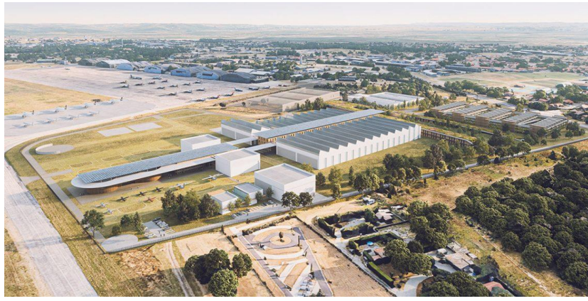
Current Infrastructure of Aura Aero
